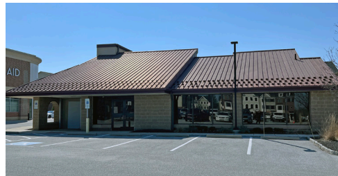
C&N's Chesterbrook office will replace our Paoli location this summer.
